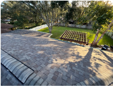
East Facing Roof
