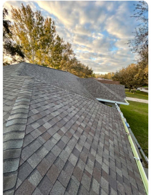
West Facing Roof
