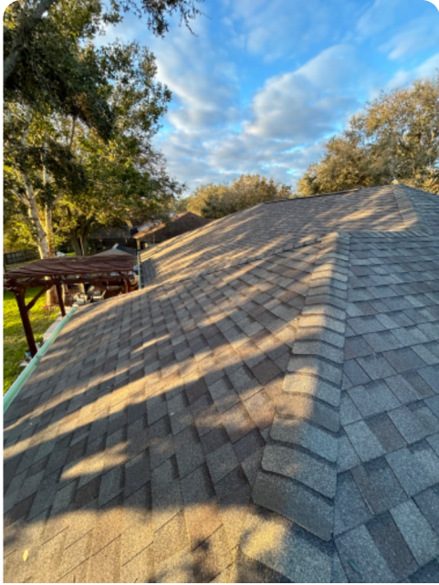
East Facing Roof
