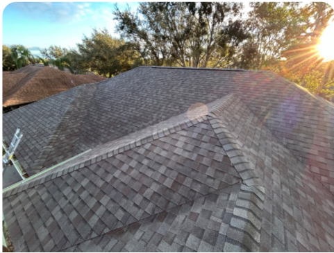
West Facing Roof
