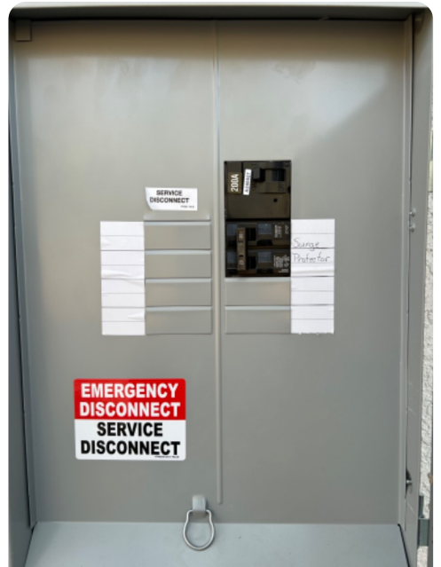
Exterior Service Disconnect
