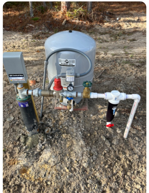
Well Pump and Main Shut Off
